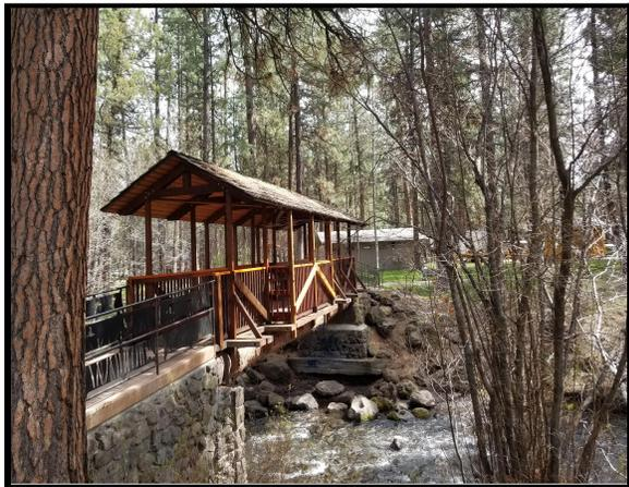
Image 3: Creekside pedestrian bridge with shake shingles and heavy timbers.
